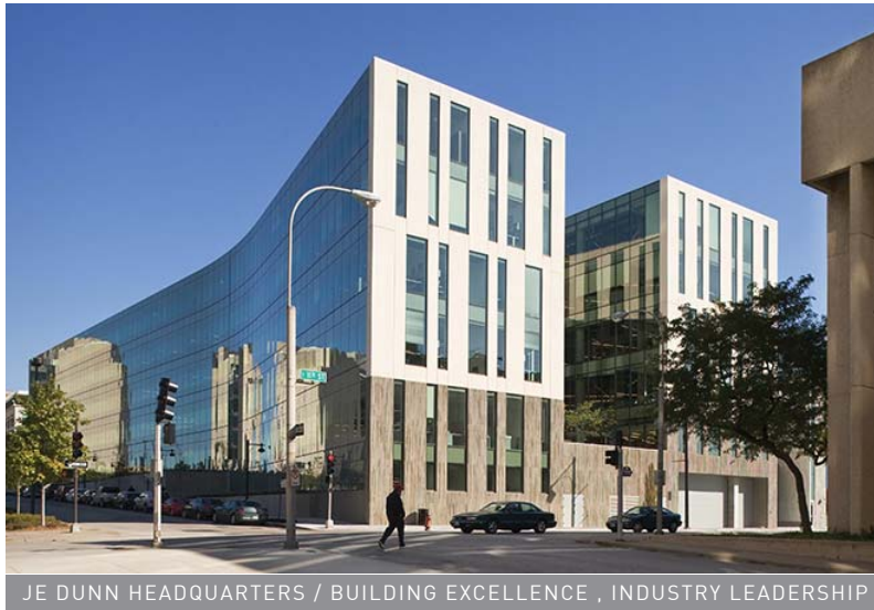
JE DUNN HEADQUARTERS / BUILDING EXCELLENCE , INDUSTRY LEADERSHIP
