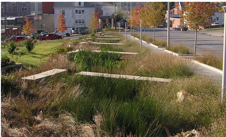
BMP STRATEGIES HOLD ALMOST ALL STORM WATER RUNOFF ON SITE
