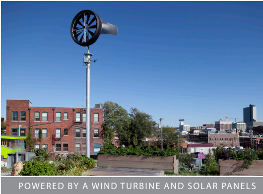
POWERED BY A WIND TURBINE AND SOLAR PANELS
